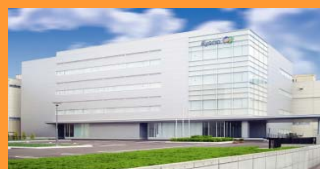
Inami plant (Toyama)
