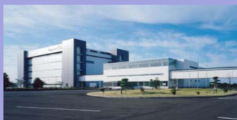
Noshiro plant (Akita)
