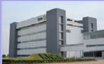
Noshiro plant (Akita)
