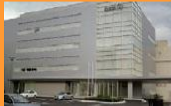
Inami plant (Toyama)
