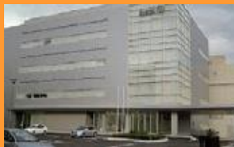
Inami plant (Toyama)
