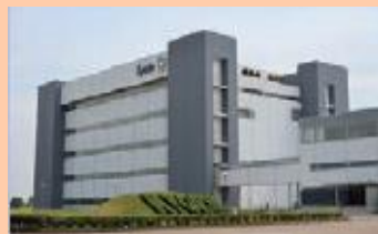
Noshiro plant (Akita)
