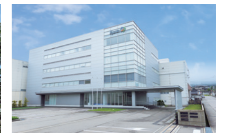
Inami Plant Location: Nanto, Toyama
