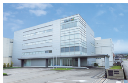
Inami Plant Location: Nanto, Toyama
